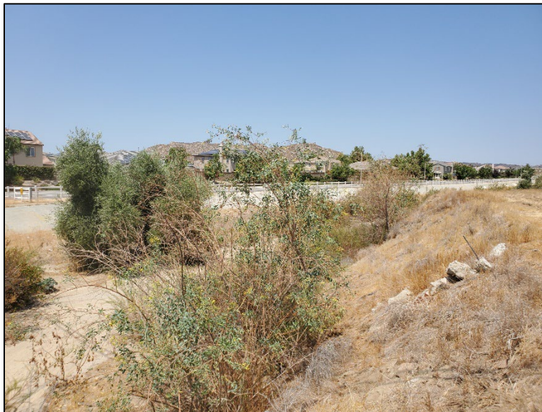
Figure 19. Representative photo of drain system, berm, and vegetation, view northwest
