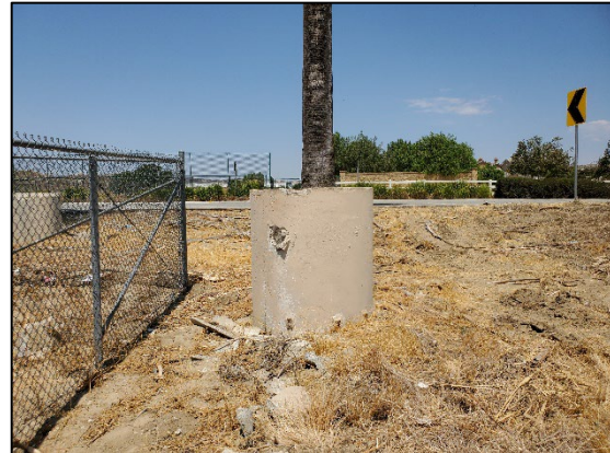
Figure 10. Feature 5, view north
