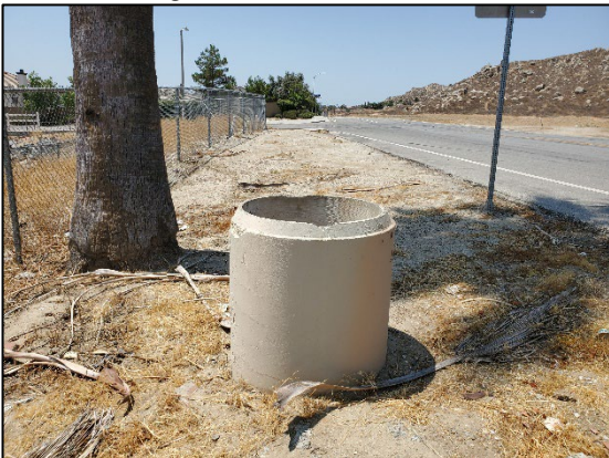
Figure 11. Feature 5, view north
