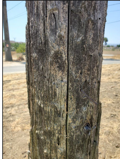
Figure 8. Feature 3, view north
