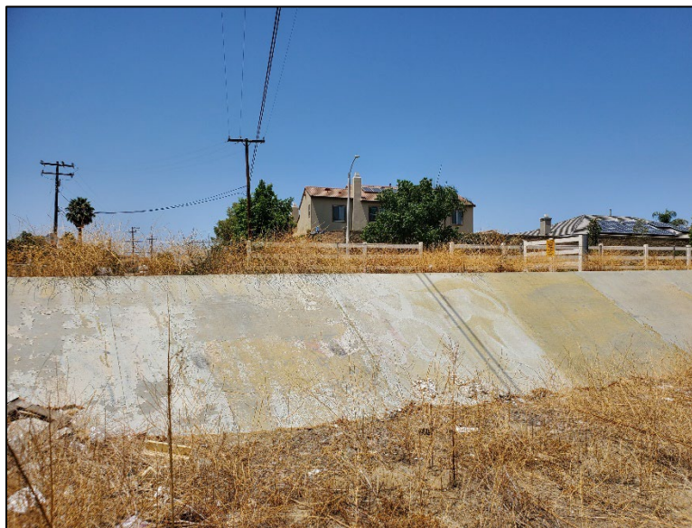
Figure 17. Representative photograph of concrete drain system, view west
